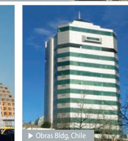
▶ Obras Bldg, Chile
